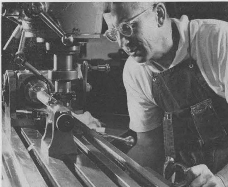
MILLING OPERATION performed here by Ted Siegrist shapes the first stage of the rocket. Special form milling cutter required for this operation was designed and built in the Development Shops. Tiniest flaw or misalignment will make piece useless.
